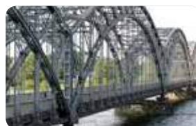
Stahlindustrie | Steel industry
